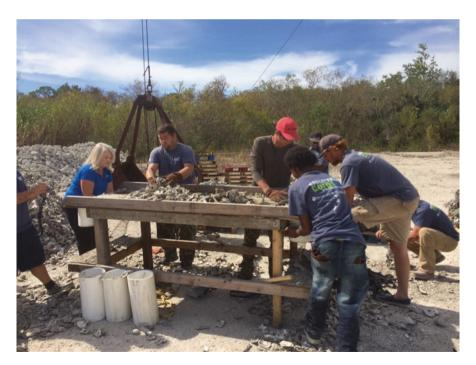
Fig. 18.5 The Conservation Corps of the Forgotten Coast in Apalachicola, Florida bagging oyster shells to be used in a living shoreline. (Photo: Holden Foley)
