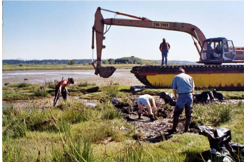
Figure 6 Swamp Excavator (photo by Pat Lim).
