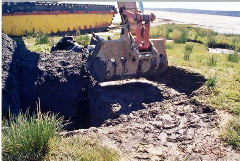
Figure 7 Excavator burying Spartina anglica (photo by Pat Lim).
