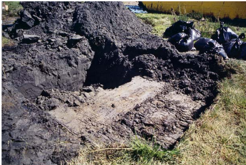
Figure 8 Excavator refilling the holes (photo by Pat Lim).
