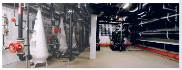
Steel cones used for adding  $CO_2$  to acidification experiments at the Matre Research Station. The pipes to the right distribute water to the research halls.
