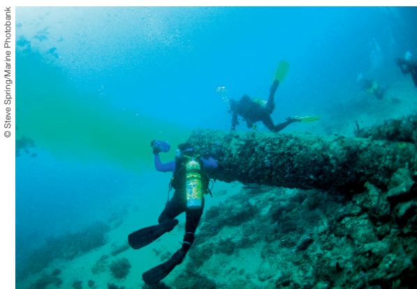
Figure 2.4. Sewage outfall discharges 15-20 million gallons of sewage upcurrent of a coral reef
