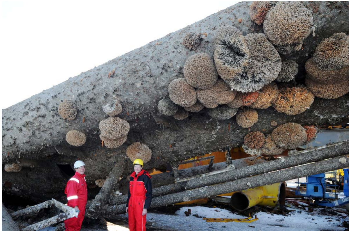
Figure 9. Lophelia pertusa colonies on the legs of the Frigg platform, decommissioned in March 2010, after 30 years in the sea (photograph: Erling Svensen).
